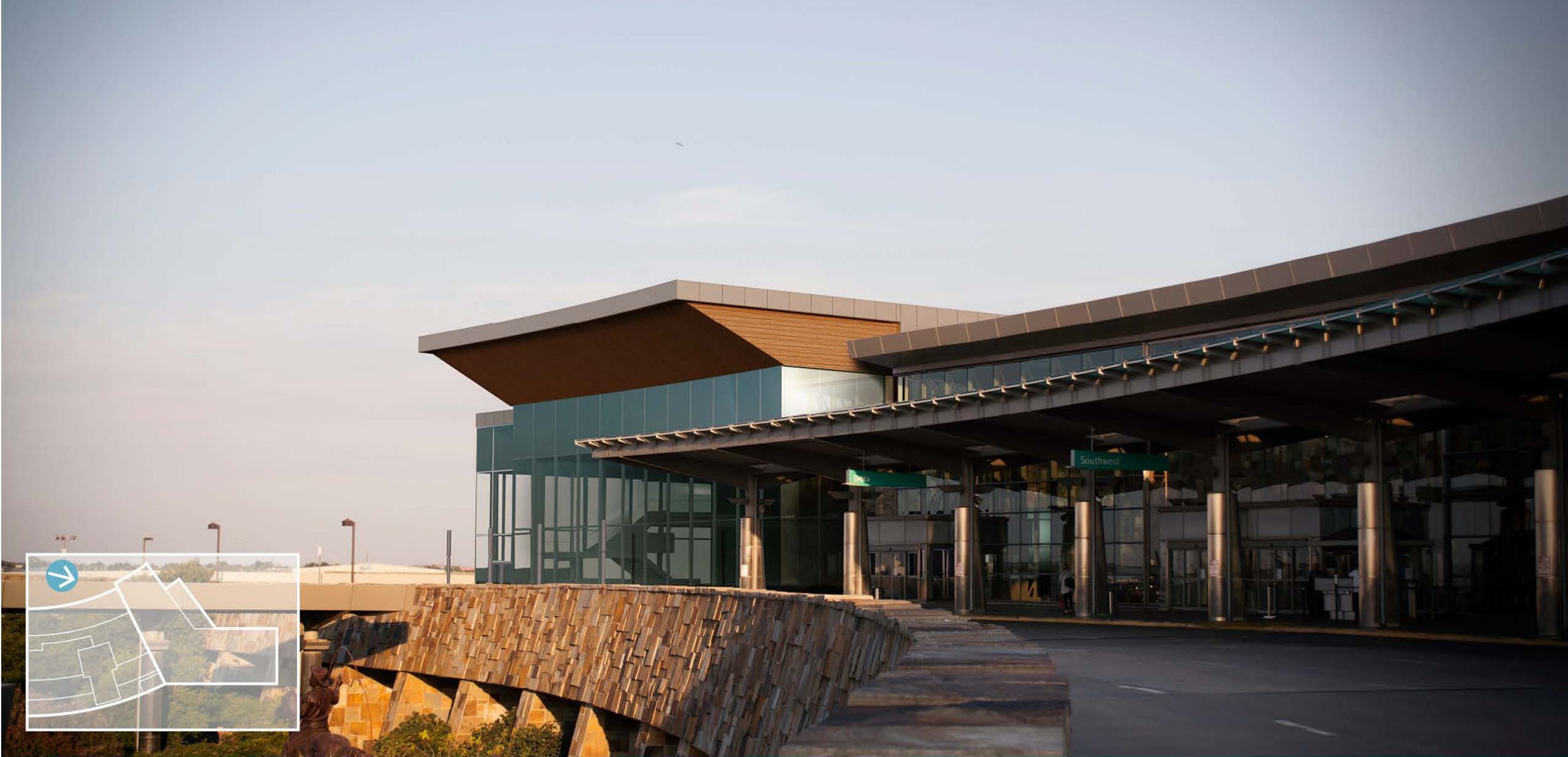
NEW DEPARTURES HALL - LOOKING EAST
