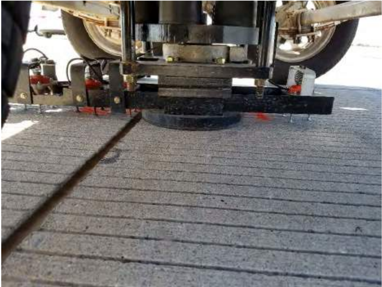
Photo 1 – Typical FWD Tests at PCC Joint Upstream for LTE Evaluation
