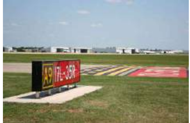
Airfield Signage and Holding Position Markings
